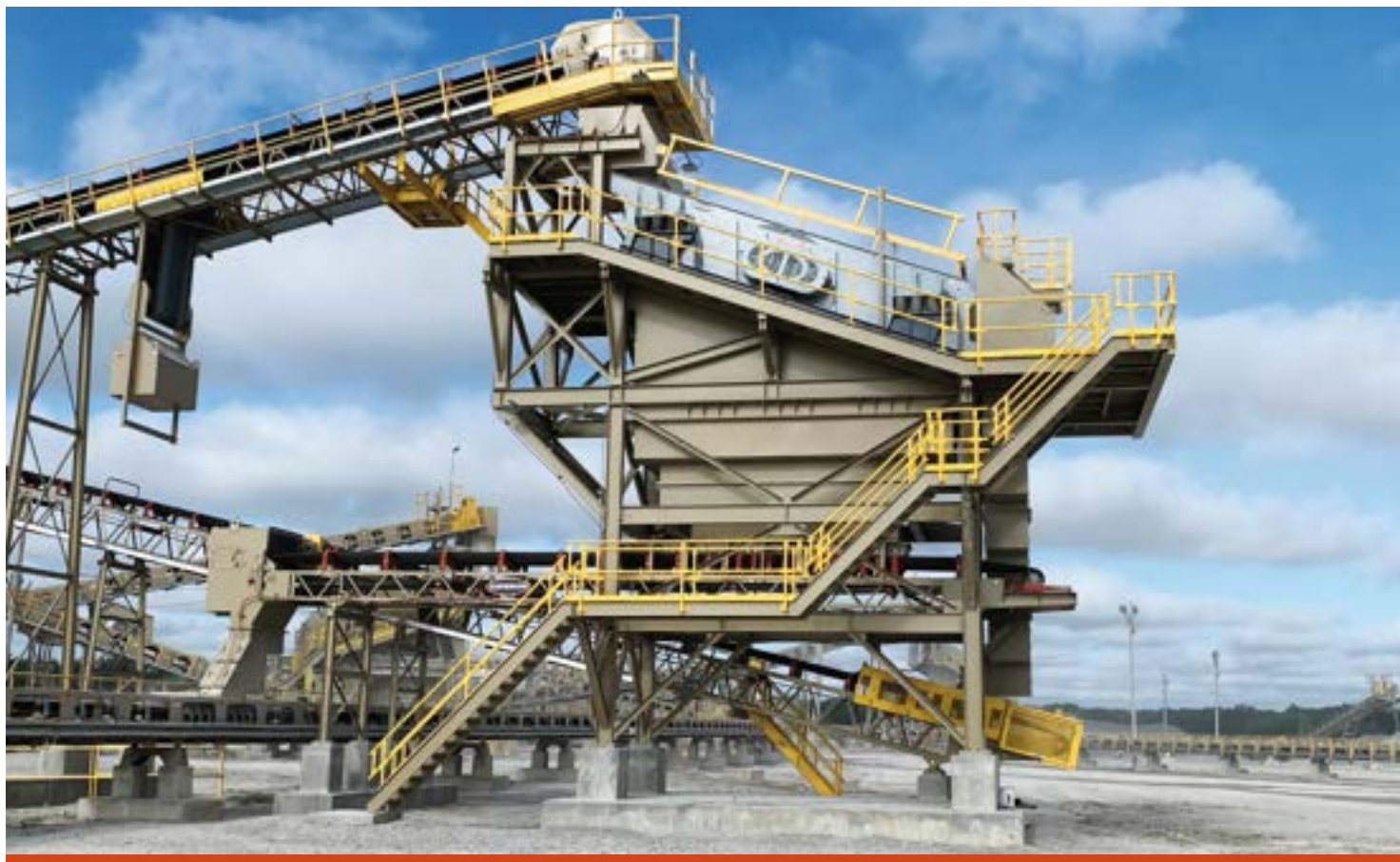
Pictured is a Superior S18242 Anthem Inclined Screen mounted on a Superior custom structure and conveyor.
