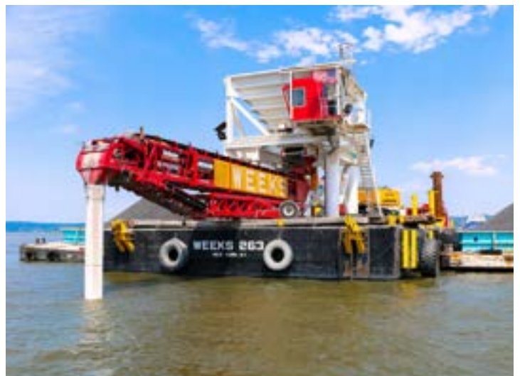
BARGE UNLOADING / DREDGE CAPPING
