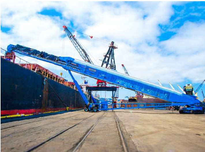
SHIP OR BARGE LOADING
